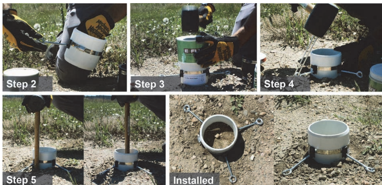
Figure 2. In-ground Receiver Installation (Steps 2-5)
